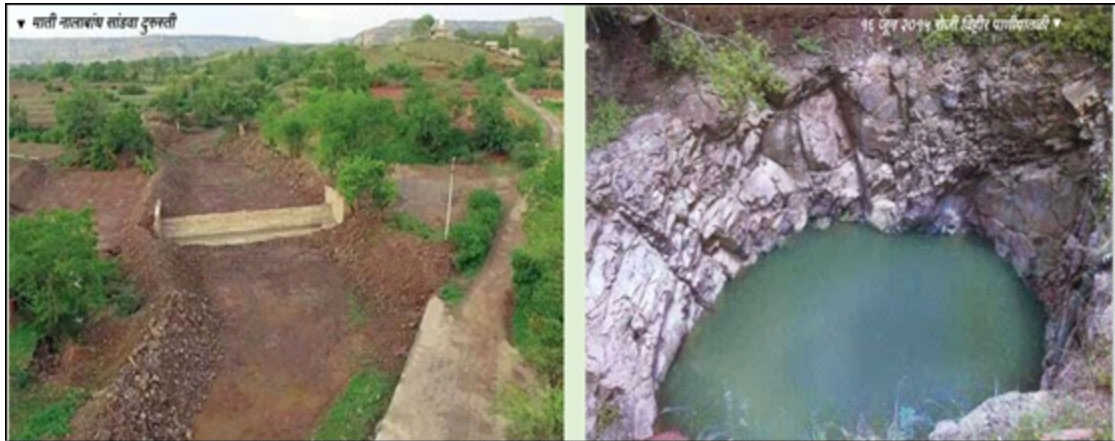
Photo: 5 Check Dam & Recharge Dug Wells (Source - 'JalyuktShivarAbhiyan' Report - 2016)
