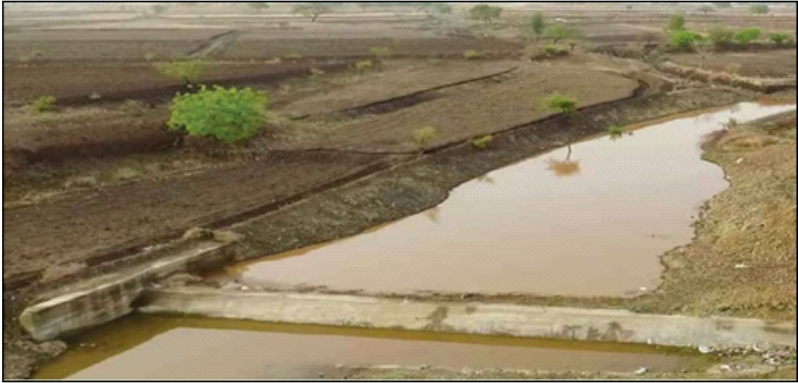
Photo: 2 Cement Check Dam at Inchbav Village (Man)
